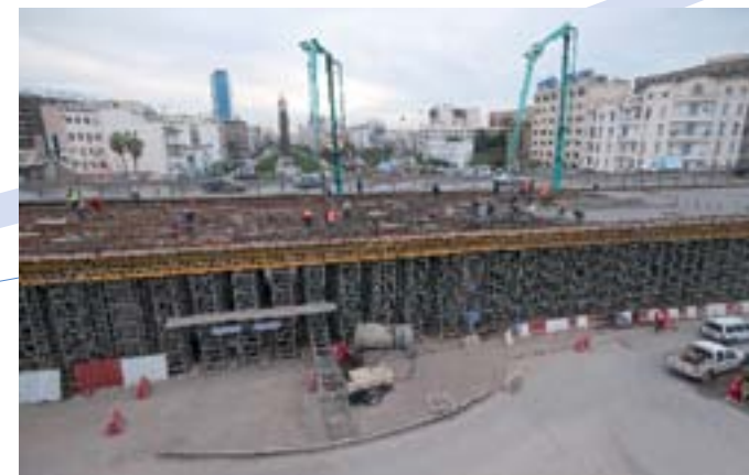
Interchange Z4 in the Republic Avenue in Tunis Prestressed concrete deck works
