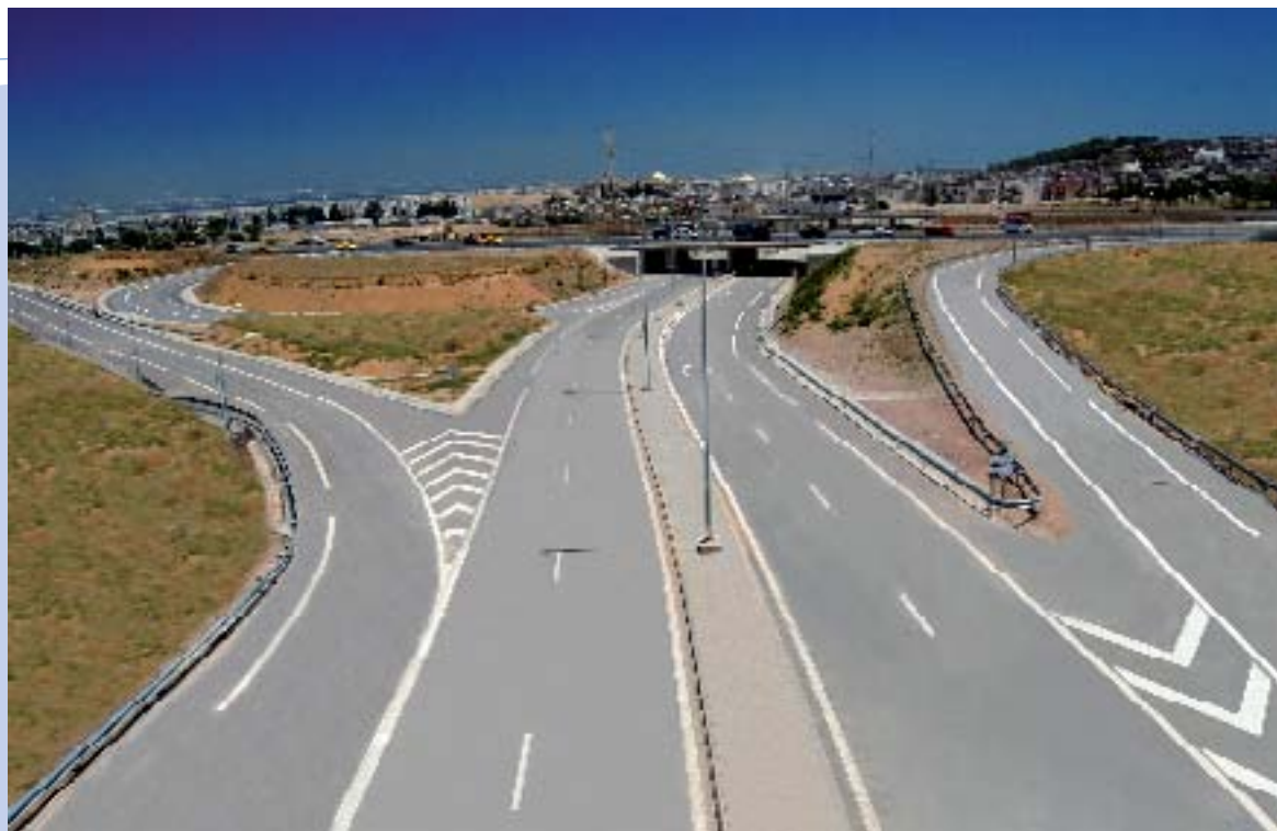
Development work of the inter-communal linking the south exit to the west exit of the capital Tunis, year 2005
